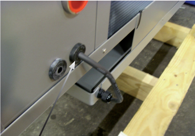
Connection cable mounted.
